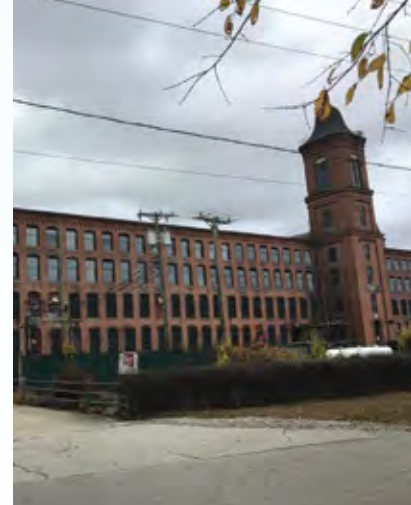
River Mill Redevelopment
